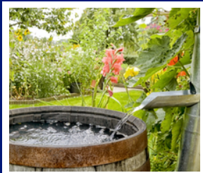
Downspout connected to rain barrel; source: prairielandsgcd.org
